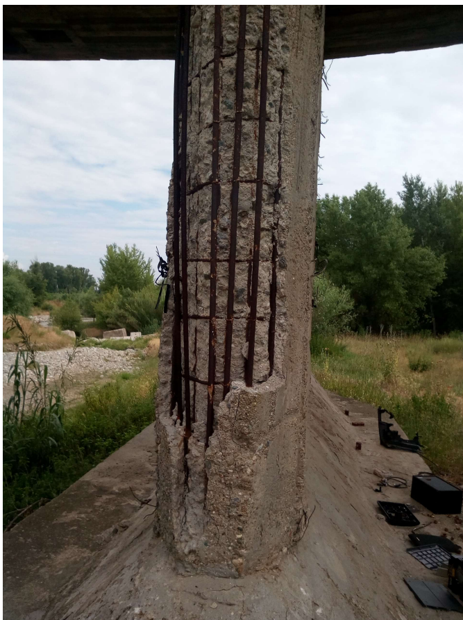
Figura 4. Pila in c.a. degradata
